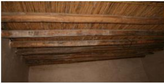
Figure 6. Wooden planked ceilings (Akram and Franco, 2016).
