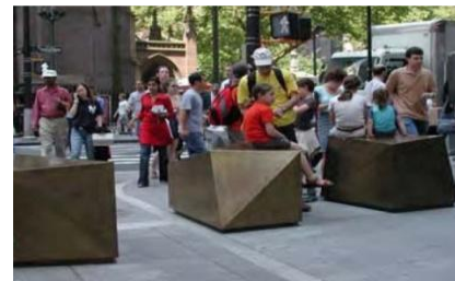
Figure 6. Up: sculptural forms, furniture and bollards serving as restrictive elements. San Francisco Federal Building (FEMA, 2007); middle: Times Square Tower, down: Wall Street, New York City, Rogers Marvel Architects (Phifer, 2005; FEMA, 2007)
