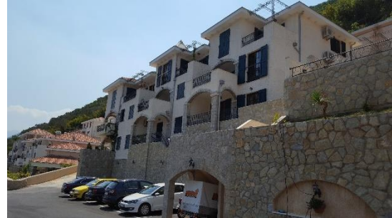
Figure 9. Excessive height of the new building and the retaining walls (Source: Kosara Kujundzic)
