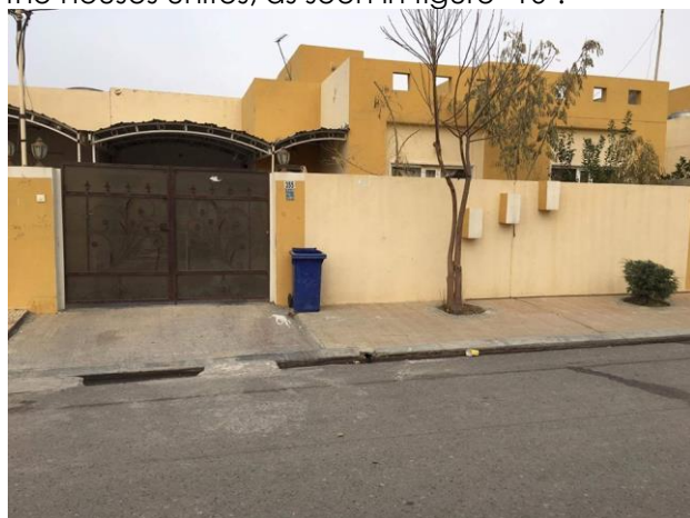
Figure 10. The frontage garden (green area) in the houses at Aarshum project. (By Author)
