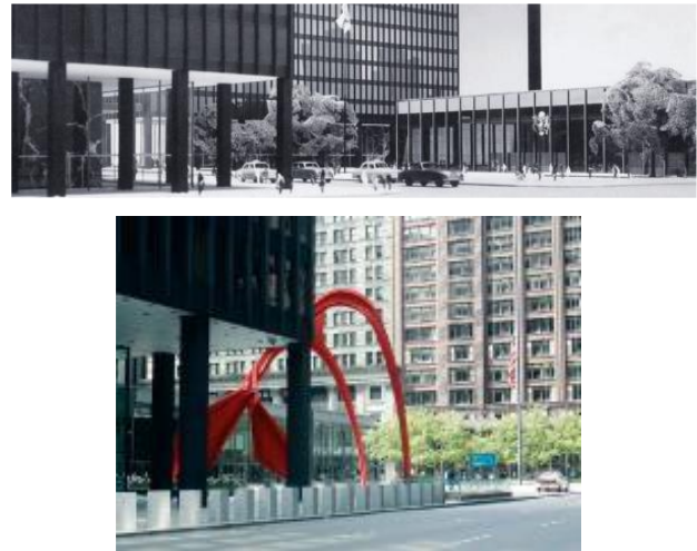
Figure 4. Security protection has been designed in harmony with the architectural identity of the building. The Federal Complex containing the three iconic buildings of Mies van der Rohe and the statue of Alexander Calder (Chicago, Illinois) (Photo General services administration by teng and associates, Chicago) (FEMA, 2007).
