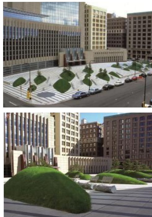
Figure 5. The Minneapolis courthouse plaza. Small lawn hills and logs prevent possible vehicle attacks along the facade of the building (FEMA, 2007)
