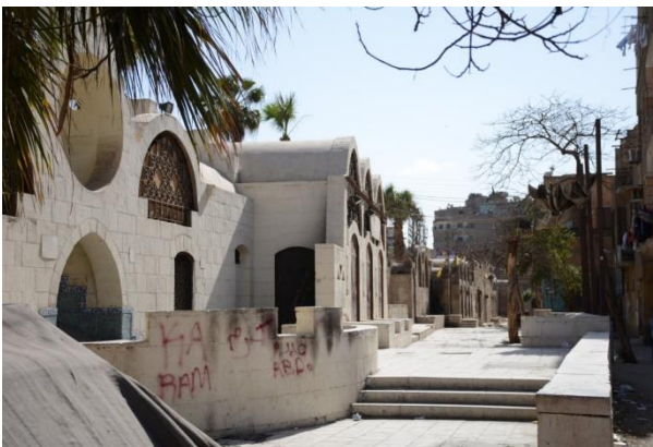
Figure 10: View from Abu-ElDahab Street Entrance, Authors, 2018.
