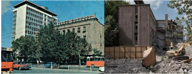
Figure 4: The Bank of Municipalities building in 1970's (Sözen, 1984) and in June 17 th of 2017 (Interpress)
