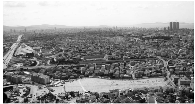
Figure 2: Current Structure in Fikirtepe
